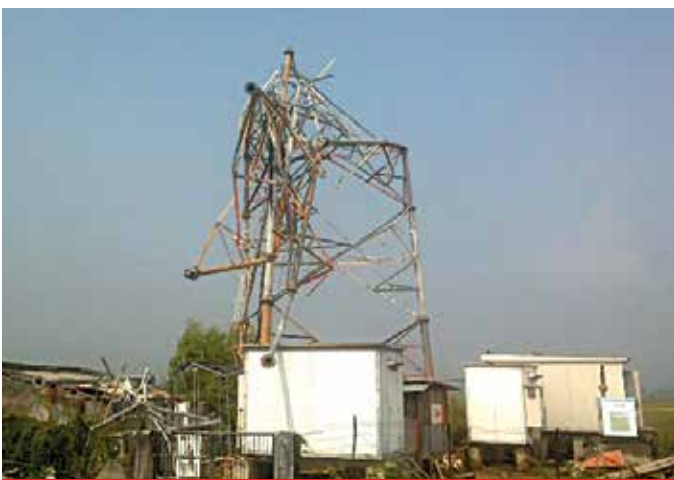
Balipadar tower site in Odisha after collapse (above) and after restoration (below)
